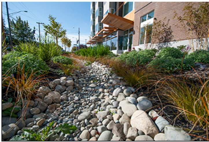
[enlarge] A bioswale along South McClellan Street filters rainwater from the alley and street.
